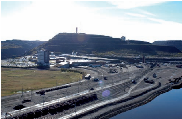
View of Kiirunavaara. LKAB has been mining iron ore for more than 100 years. In the beginning, the mining was open cast, above ground; it wasn't until the 1960s that the mining went underground.
